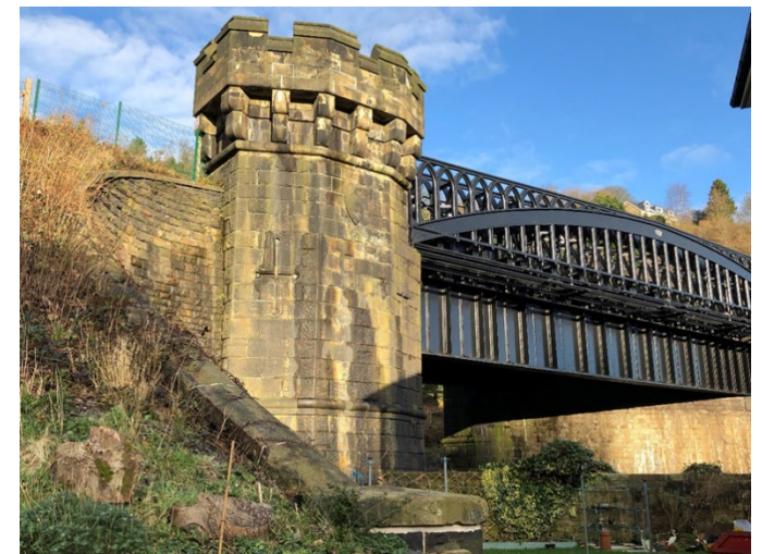
Gauxholme Railway Bridge in Shade – grade 2 listed
