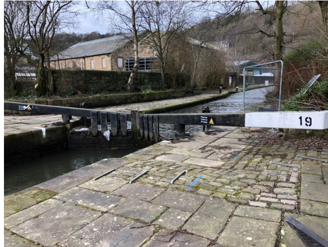
Lock 19 of Rochdale Canal near Rochdale Road – grade 2 listed
