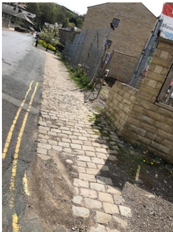
Stone Setts at Key Sike Lane
