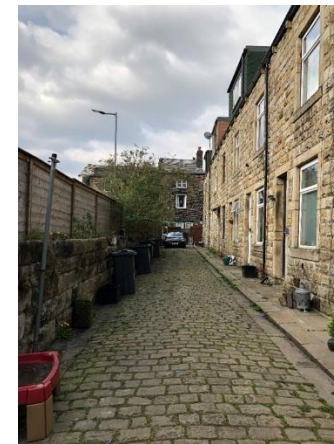
Stone Setts at Back Der Street
