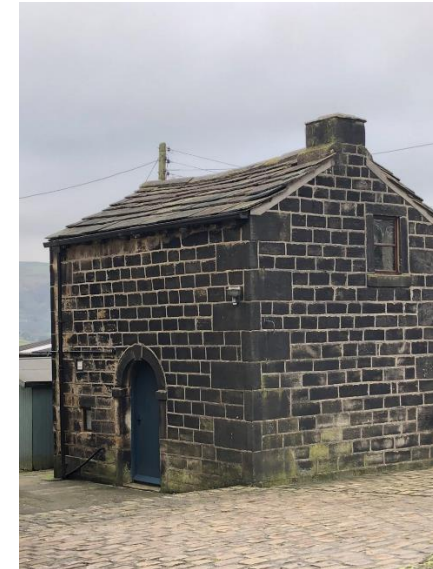
A separate building belonging to Fielden House
