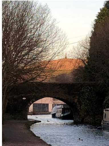
View of Stack Hills Bridge – grade 2 listed with Stoodley Pike in the distance
