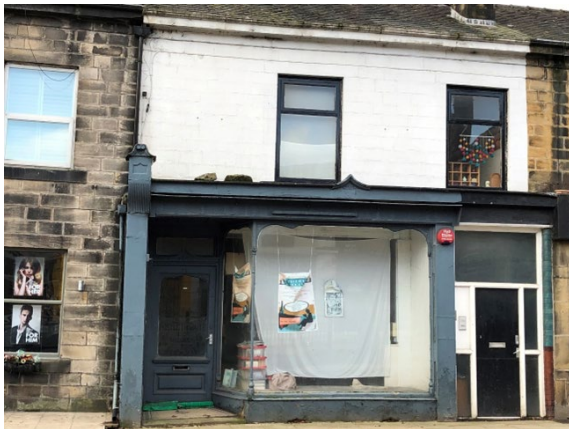
75 Burnley Road. This is the fourth in a row of stone-built shops. This one has a traditional large shop window and inset door. The wooden carved surround is traditionally Victorian.
