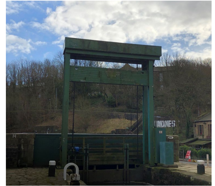
Lock 20 of Rochdale Canal near Rochdale Road – grade 2 listed
