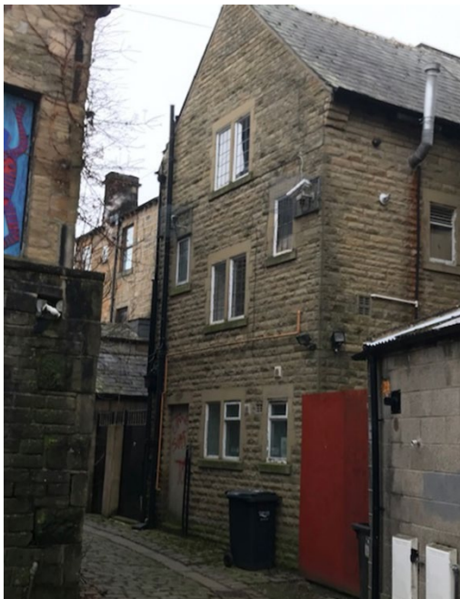
Back of 32-34 Burnley Road (formerly Fox and Goose pub) on Coupland St with cobbled street
