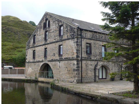
Gauxholme Warehouse – Grade 2 listed
