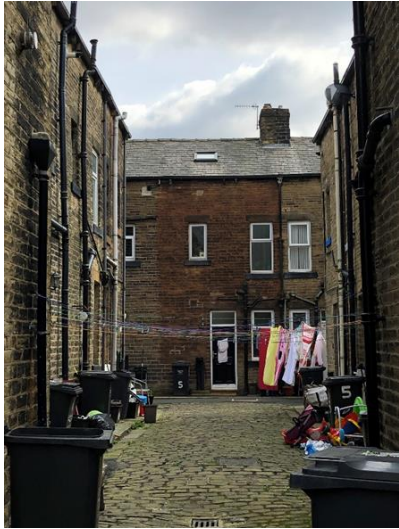
A cobbled alleyway next to Hope Buildings
