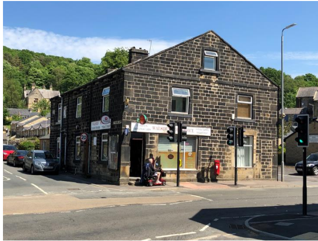
The Post Office on the junction of Rochdale Road and Hollins Road
